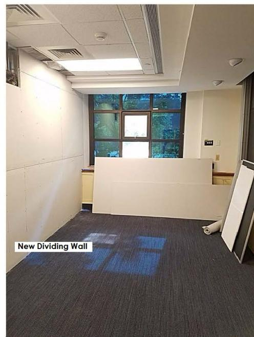
*Figure 3: Exterior Foam Board, 1075 Side (L), New Dividing Wall, 1077 Side(R)*
