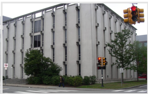
Engineering and Science Laboratory Building 58 Oxford Street Cambridge, MA
