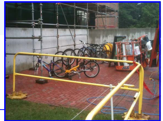
Bike Racks at Oxford Street Entrance Photo: Harvard Green Building Services, 2010
