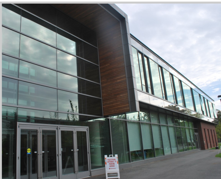
Northwest Labs Photo: Harvard Green Building Services, 2009
