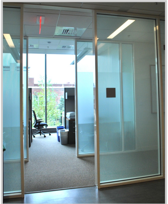
East Wing Offices Photo: Harvard Green Building Services, 2009
