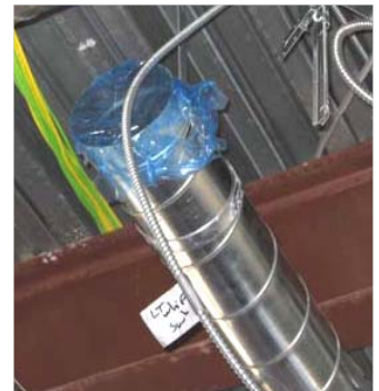
HVAC Protection Ductwork was sealed during installation
