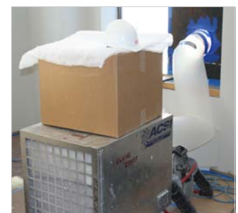
Pathway Interruption Exhaust filtered & directed outside
