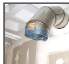
IAQ Management HVAC Protection: Ductwork kept sealed before installation
