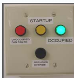
Indicator Panel Green Light means it is safe to work in the Lab
