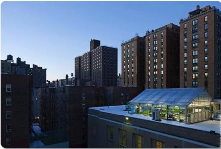
Rooftop greenhouse on a NYC public school. Source: http://www.farmxchange.org/top-8-urban-farms-in-the-world/
